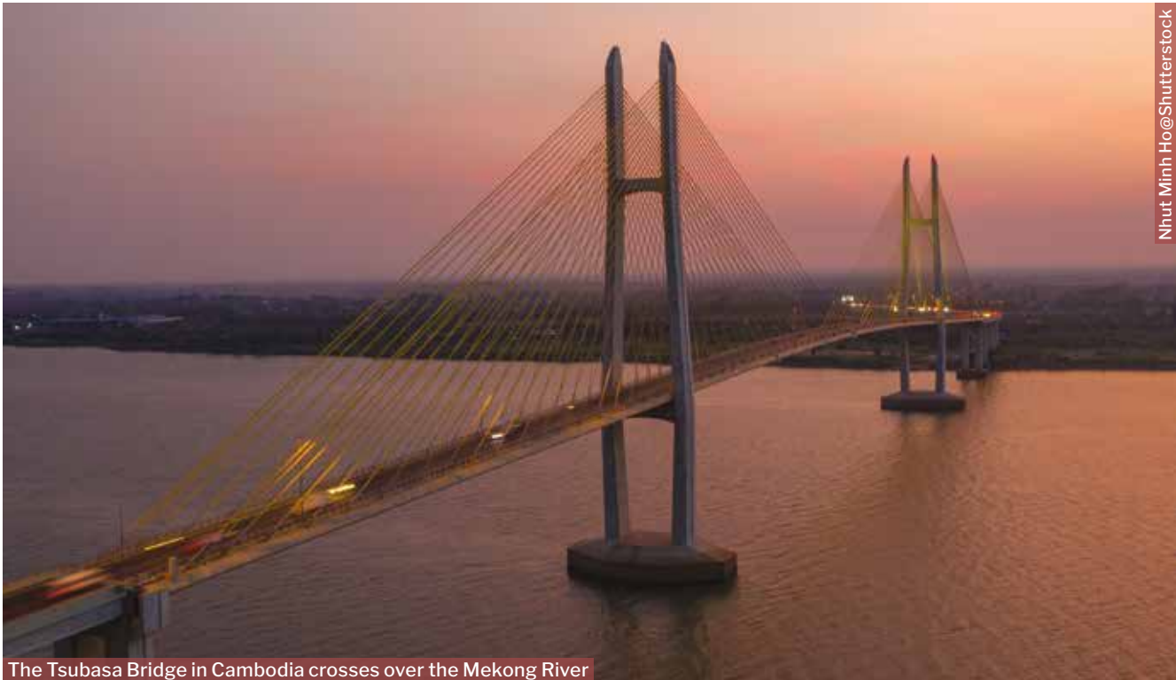
The Tsubasa Bridge in Cambodia crosses over the Mekong River
