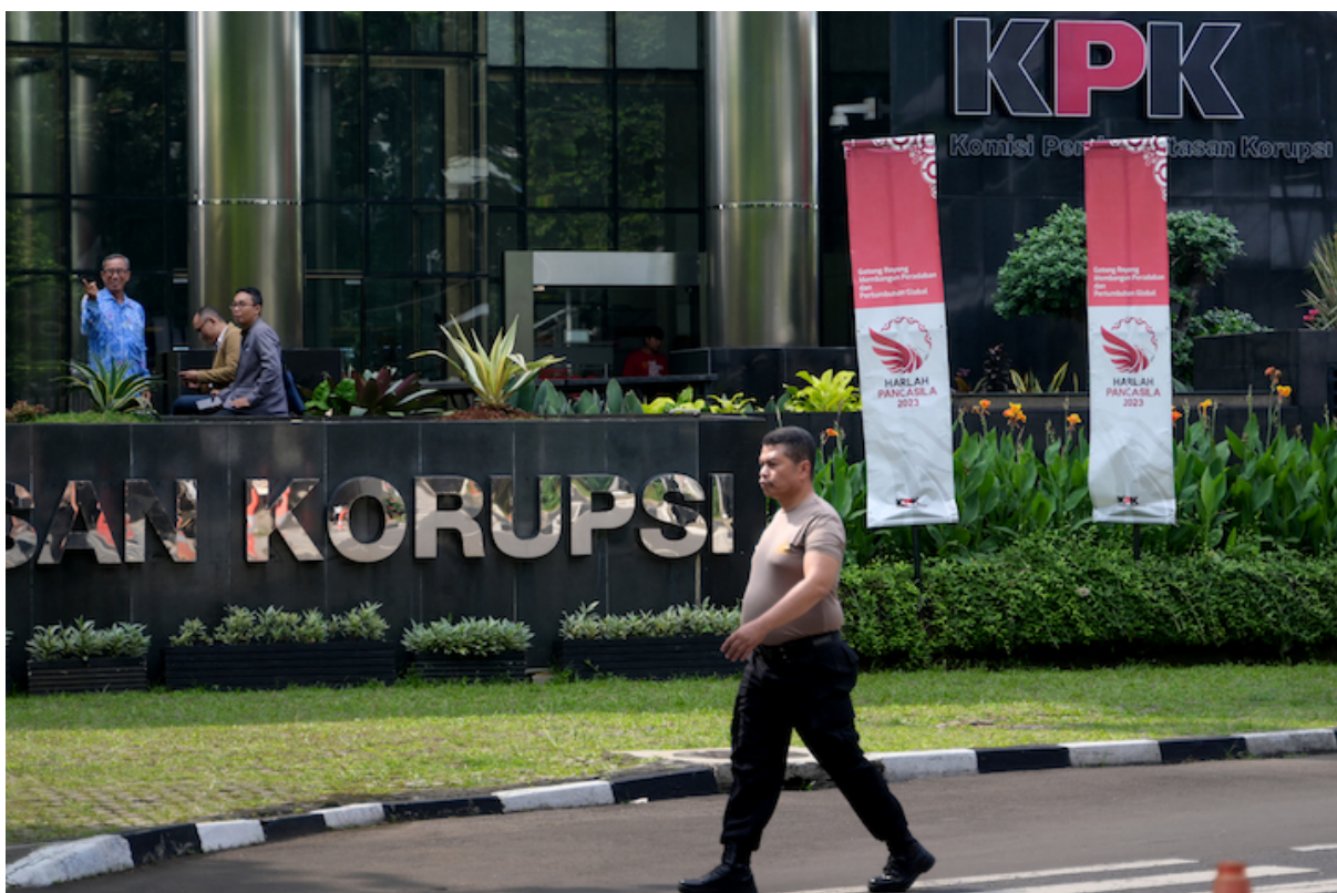
The Corruption Eradication Commission (KPK) building in Jakarta. Picture taken on 27 June 2023. (Photo by BAY ISMOYO / AFP).
